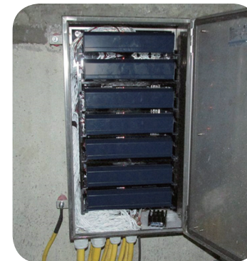
7 sets of ADL-200A laminated in Iran Dam site
