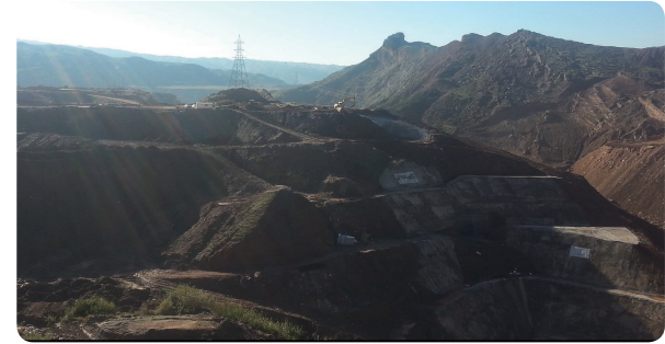
Foundation at Konjancham dam in Iran
