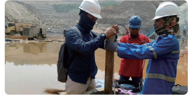
Water press at Ladongi dam in Indonesia
