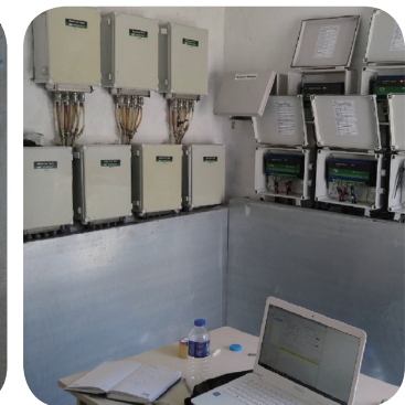
Installation in Turkey Dam site
