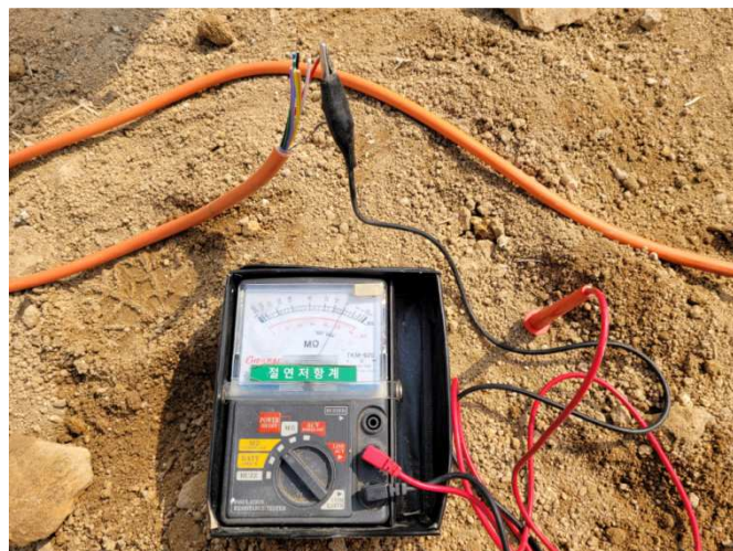
[ Insulation defect : Below 100\text{M}\Omega ]
