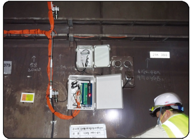
[ADL-16V Installation in tunnel]
