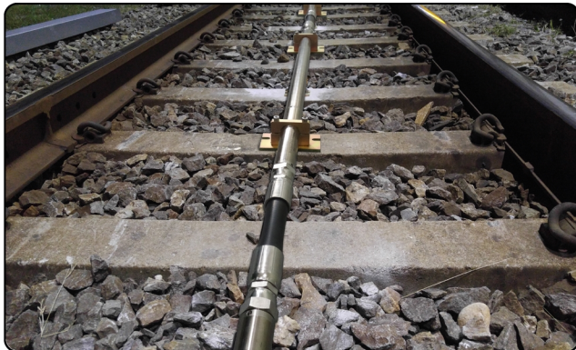
[Installation of ACE-RTM]
